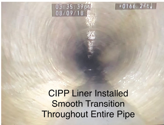
Sanitary sewer mains before (above) and after (below) liner installation.
