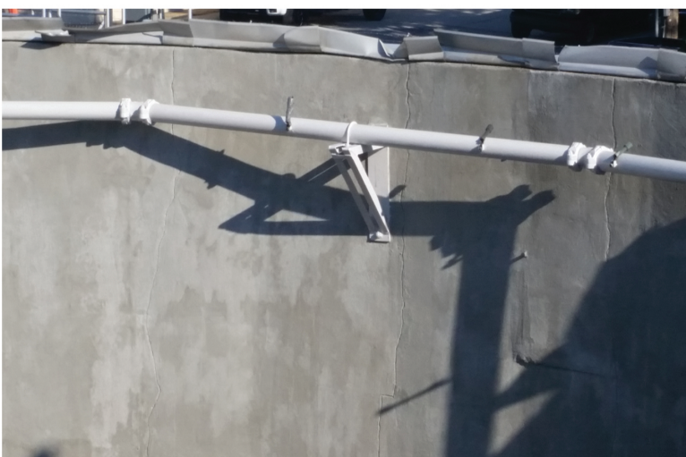
An up-close look at crack repair inside the tank.
