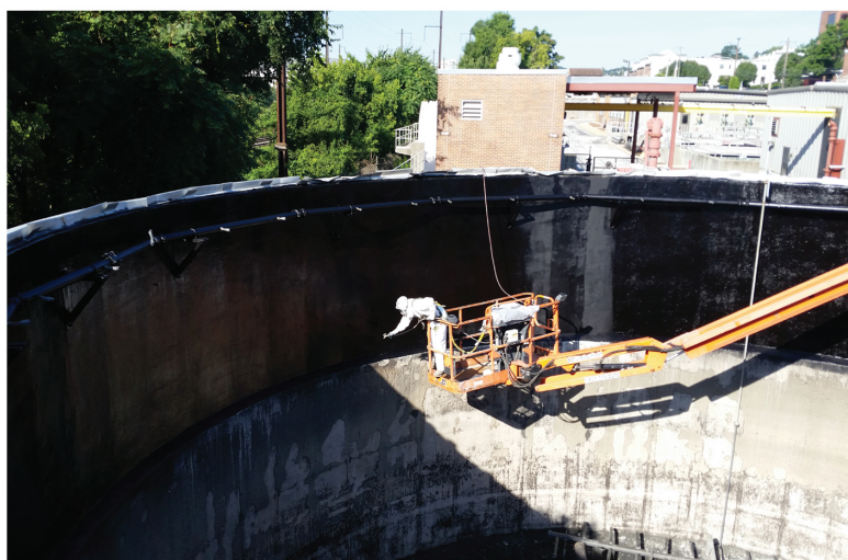
A worker applies a second application of coating.
