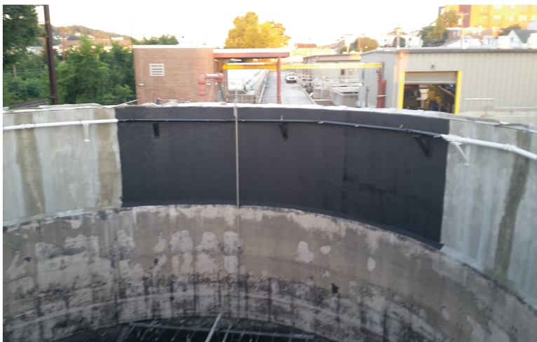
A "before" view of the empty tank where contractors are removing the old coating (top portion of tank).
