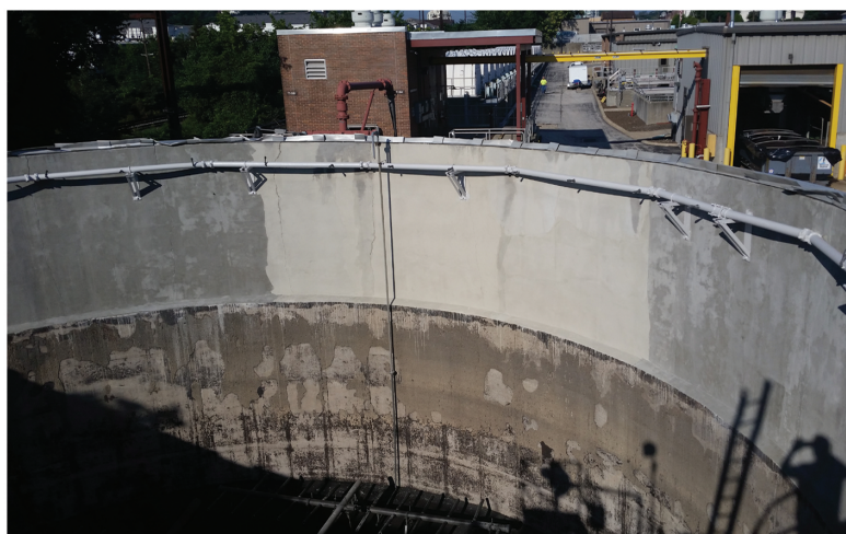
Seen here in white are portions of the tank following the cementitious coating.
